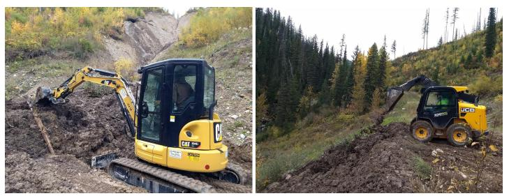
All Finished and Graded Out with a ditch to allow water to traverse the trail. Well done!
